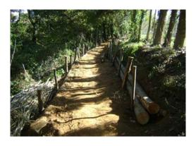
Without crossing the stakes it can also be useful in zones with slope. As we increase the front level, and unless it acts a sediment barrier, it is filling and compacting the part from the back.
