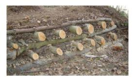
The front must not be vertical but it should have inclination in favour of the slope.
