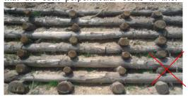
The diameter of the logs can be highly variable. We usually work with diameters of 20 to 30cm. It has to take into account that in many logs the diameter is not homogenous and must be compensate it in the construction with different diameters for keeping regular horizontal levels.
