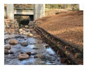
Naturalea uses wood of chestnut (slow degradation), although if it's viable, we use wood from the area. For example an acacia tree like the robinia previously treated to prevent regrowth (is an invasive aloctone plant) works very well because the wood is hard. We must be careful with the riparian vegetation or other ones like poplars and the genus *Platanus* because of their fast degradation.
