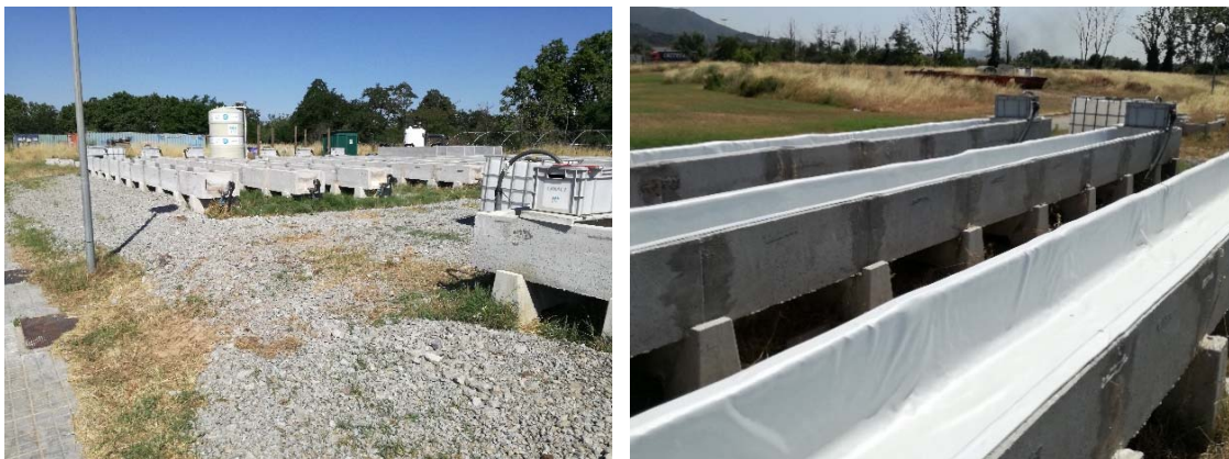
New waterproofing system for URL channels
