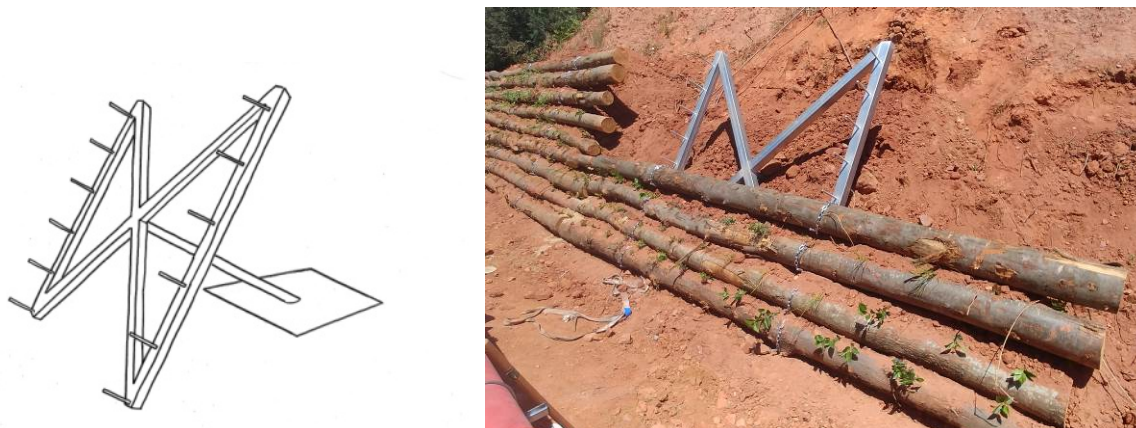
Scheme of the Loricata cribwall and image of the initial phase of the installation
