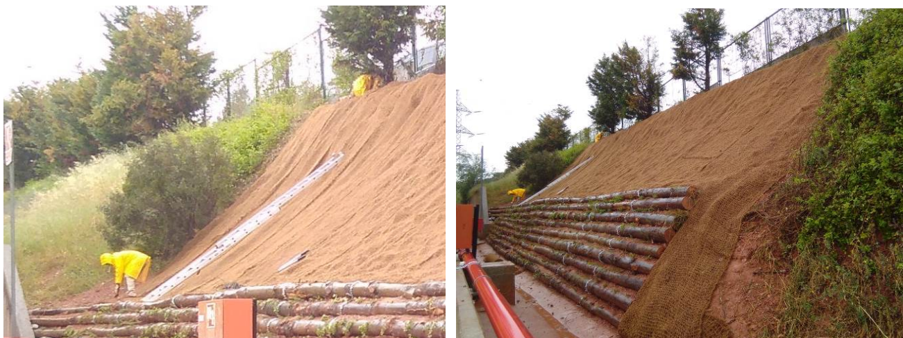
Images of the installation process of the seeding mat
