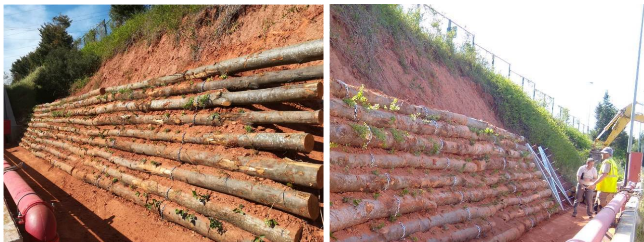
Images of the construction of the Loricata cribwall
